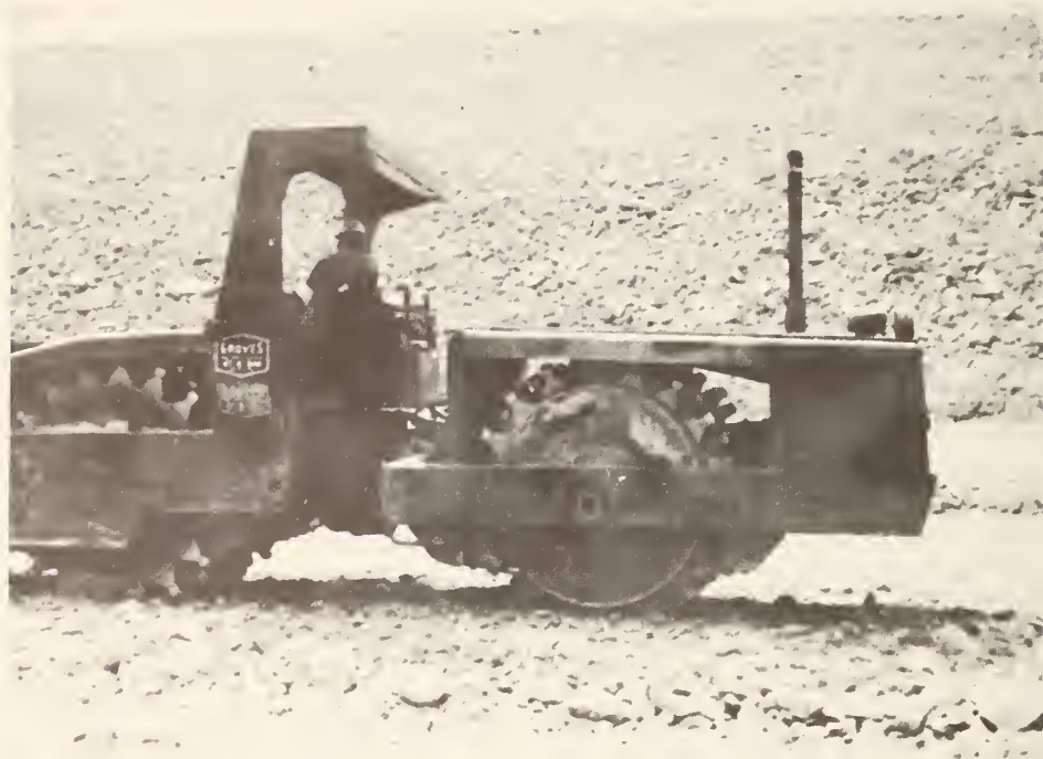
Figure 32. Heavy tamping roller with square feet
